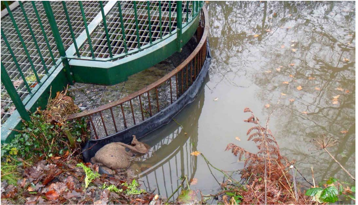
A simple piece of pond-liner sufficed as barrier fixed in place with cable-ties/wire/sand-bags
