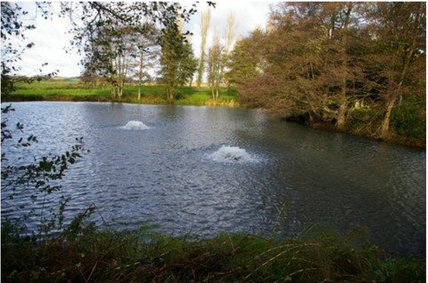
Splash pumps at Wellingham Lake ensure oxygen content in the water is high
