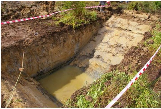
Trial pit excavation in the field north of Pond Lye car park. September 2017 (left) and December 2017 (right). Water approx. 5ft.
