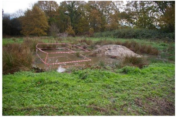
Trial pit excavation in the field north of Pond Lye car park. September 2017 (left) and December 2017 (right). Water approx. 5ft.
